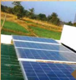
1,250 watt solar panels installed at the Foundations Community Centre in Pench. The panels supply energy to a pump and help fetch 2,100 litres of water an hour from 170 feet underground.
